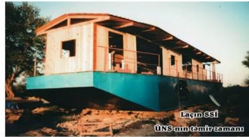
Lachin ISD - FBS during the repair
