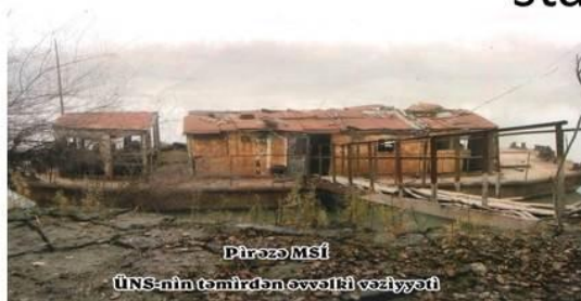
Piraza MIU - Condition of FPS before repair
