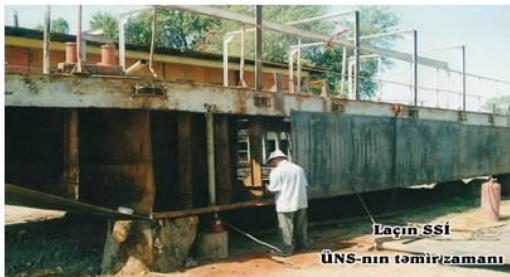
Lachin ISD - FBS during the repair
