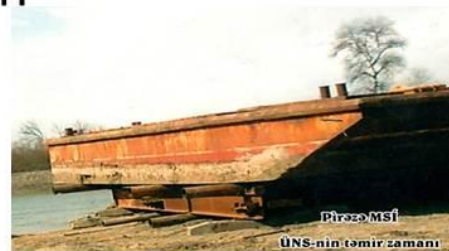
Piraza MIU - FBS during the repair
