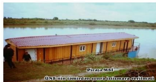
Piraza MIU - FBS operation after the repair
