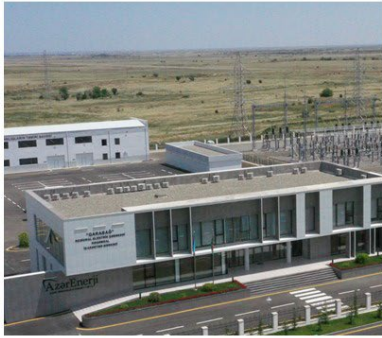
AzerEnergy Karabakh Regional Digital Control Center
